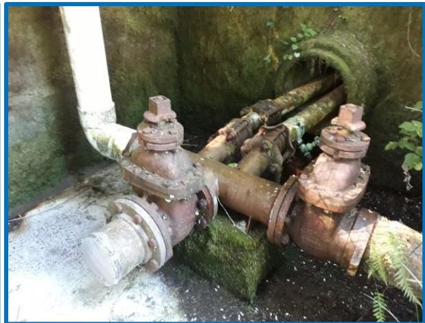
Figure 2.3: Spring #1 Manifold Valving
