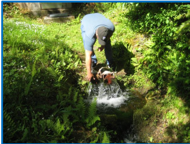
Figure 2.2: Spring #2 Overflow Pipes
